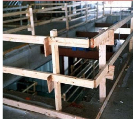
Properly installed guardrail system.
