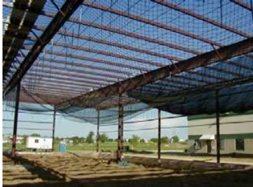
Safety nets used in construction sites.
