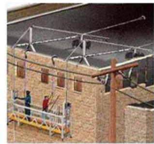
Two-point Swing Stage Scaffold
